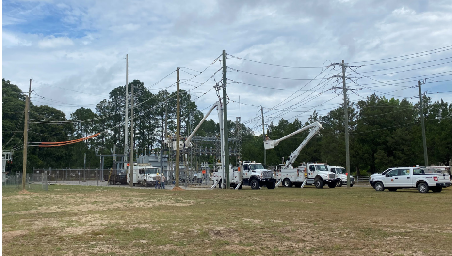
Crews perform work at the Auburn substation north of Crestview in May.
